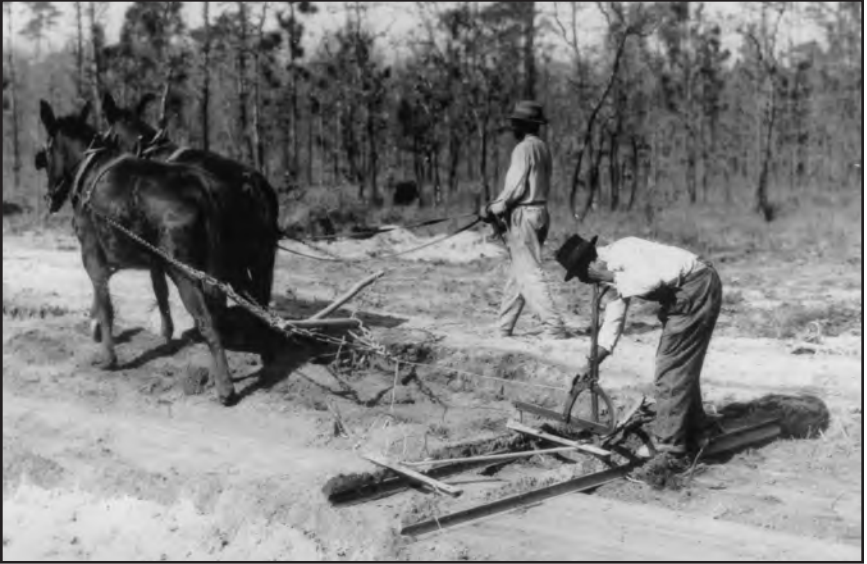
The construction of the No. 2 Course in 1901
